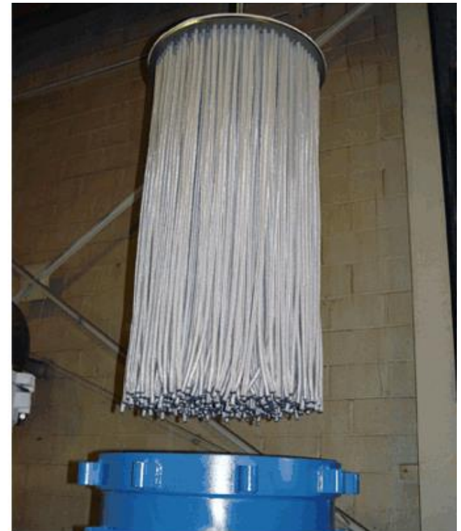
Lowering the filter tube sheet assembly into Defender
