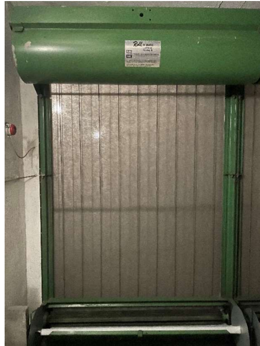
Luftfilter (Rollbandfilter)
