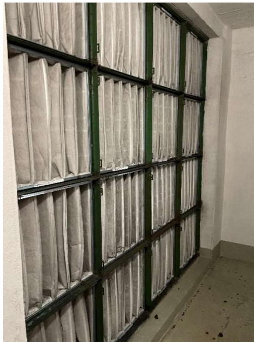
Luftfilter (Taschenfilter)
