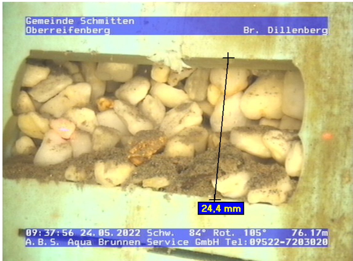
Abb. 6: gebrochene Filterstegge, lockerer unverockerter Filterkies
